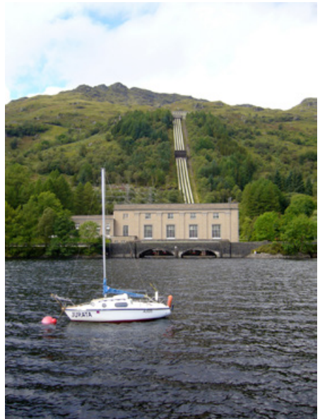
Loch Sloy HE power station
